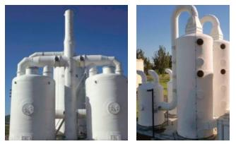
Carbon Adsorbers used as polishing units following a Biotrickling filter.
