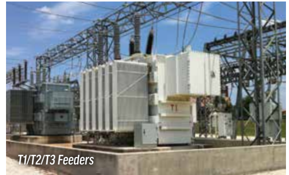
Electric Aging Infrastructure and Pole Replacements
